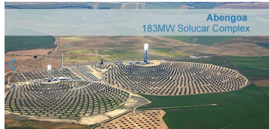
Central receiver 'power tower'
